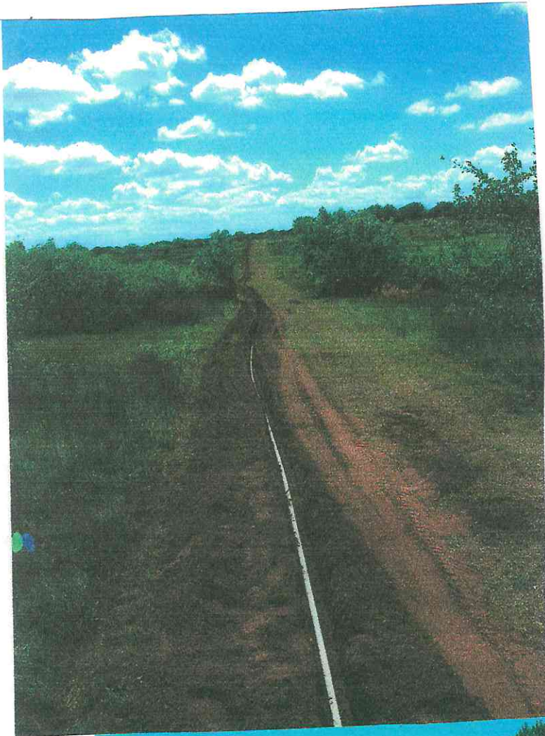
LAYING WATER LINES 2006
