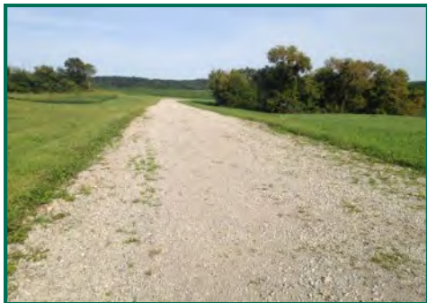
Access Road from 80th Ave. NW
