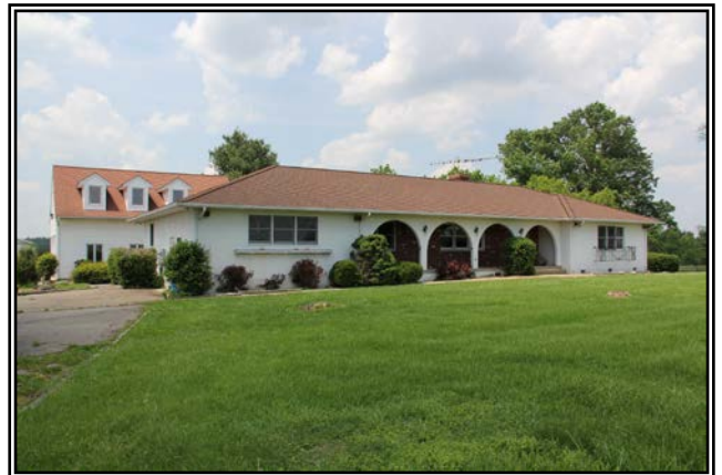
FRONT VIEW OF HOUSE & GARAGE
