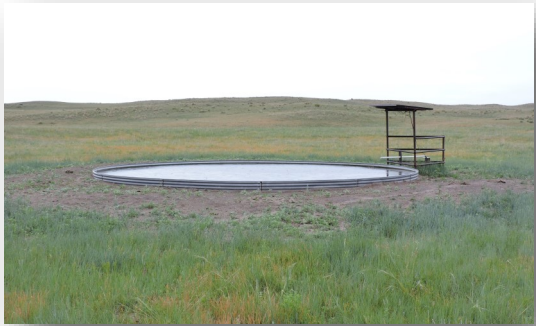
Southeast Well with Solar Panel
