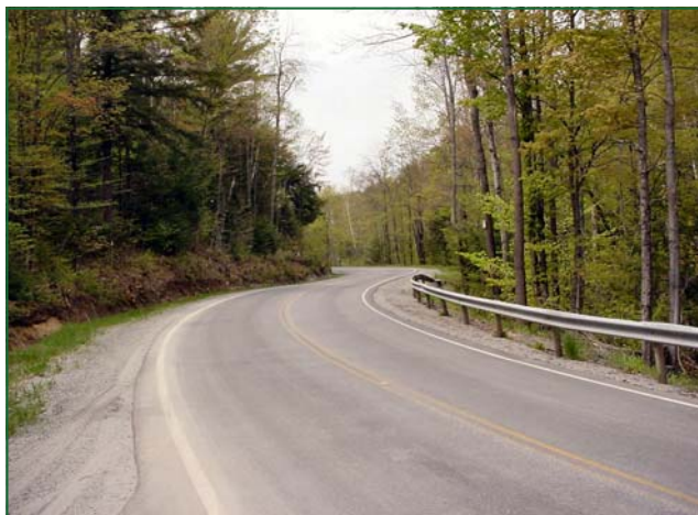
Route 4 frontage provides access and several possible driveway sites.
