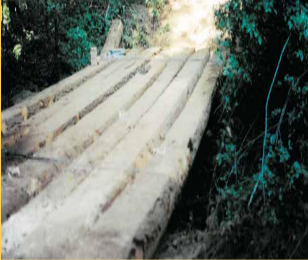
2002. Bridge under construction over Ashland Creek.
