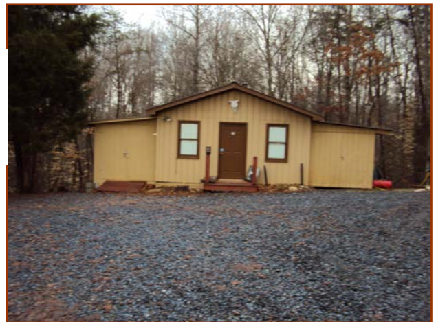
35' x 22" Metal Building with 2 attached sheds
