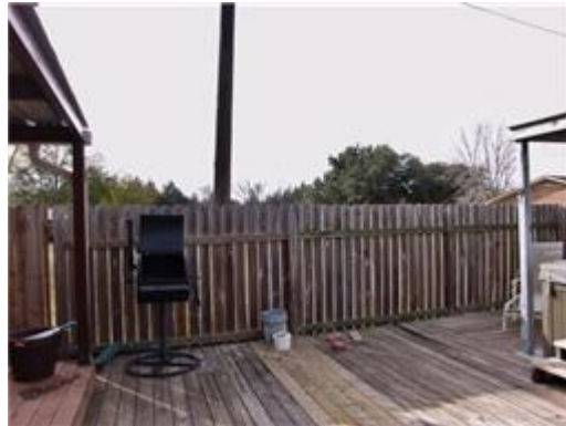
Deck - great area for grillin'
