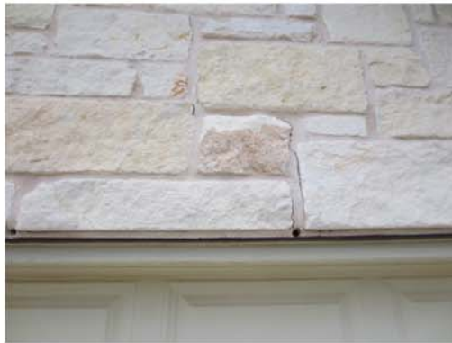
Cracks at right side of garage lintel
