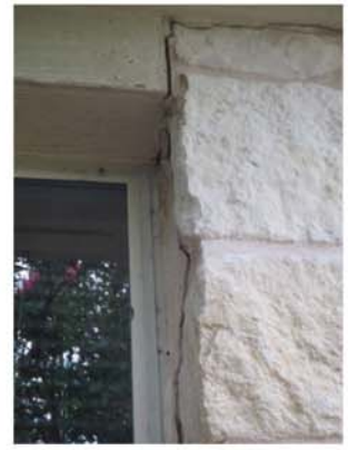
Transferrance of crack along left side front window
