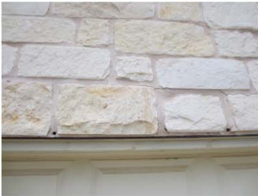
Cracks at center of header
