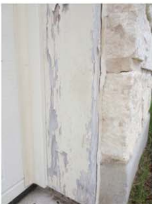
Paint deterioration at garage door trim
