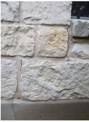
Crack at left rear window bottom
