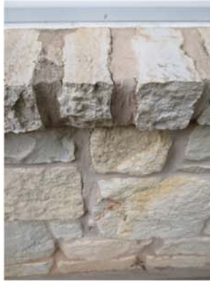
Crack at right rear window sill (center)
