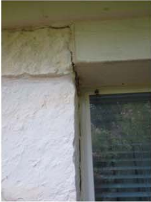
Crack at right rear window top
