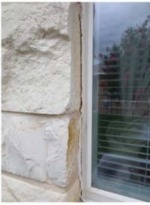
Crack at right front window edge
