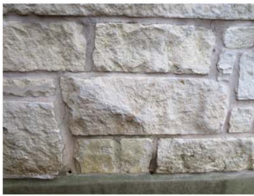
Slight cracking above fracture
