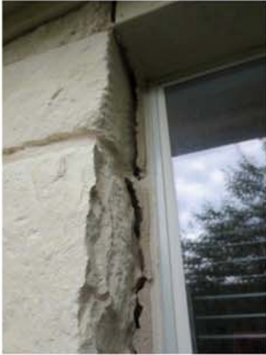
Large gap at left rear window top
