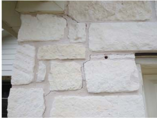
Cracks at left side of garage lintel
