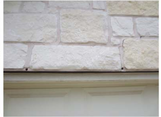
Crack at left side of garage header
