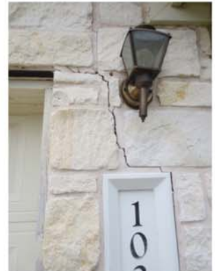
Severe crack at right side of lintel
