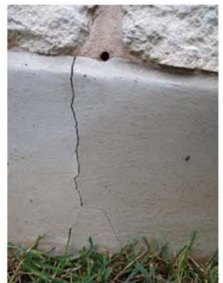
Severe crack in left rear grade beam
