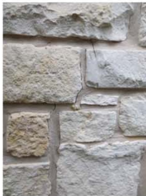
Crack at right rear wall
