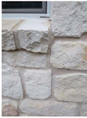
Crack at right front window sill
