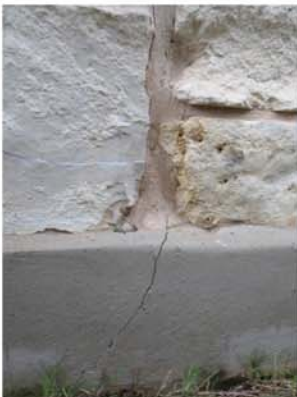
Crack in grade beam
