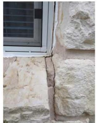
Crack at right rear window corner
