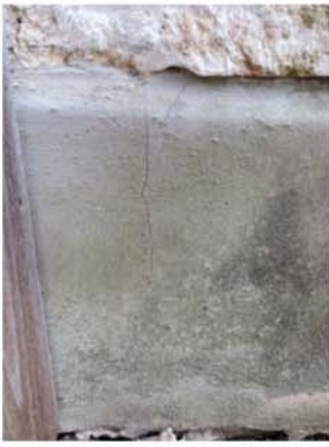
Left side front grade beam fracture
