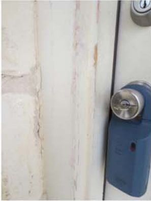
Paint deterioration at front door trim
