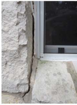
Large gap at left rear window bottom
