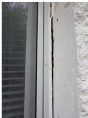
Crack at right rear window edge
