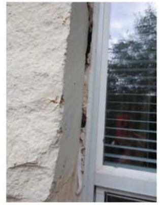
Large gap at left rear window edge
