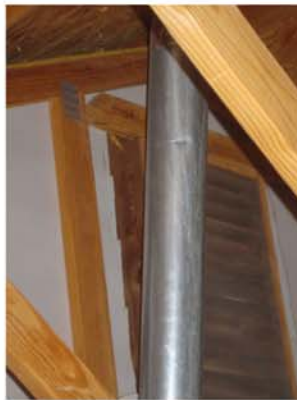
Previous water penetration at dryer vent (streaks)
