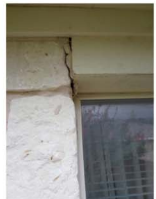
Crack at right front window top
