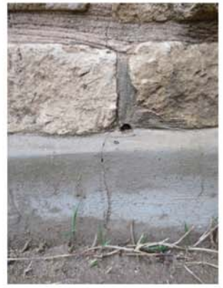
Transferrance of crack below window
