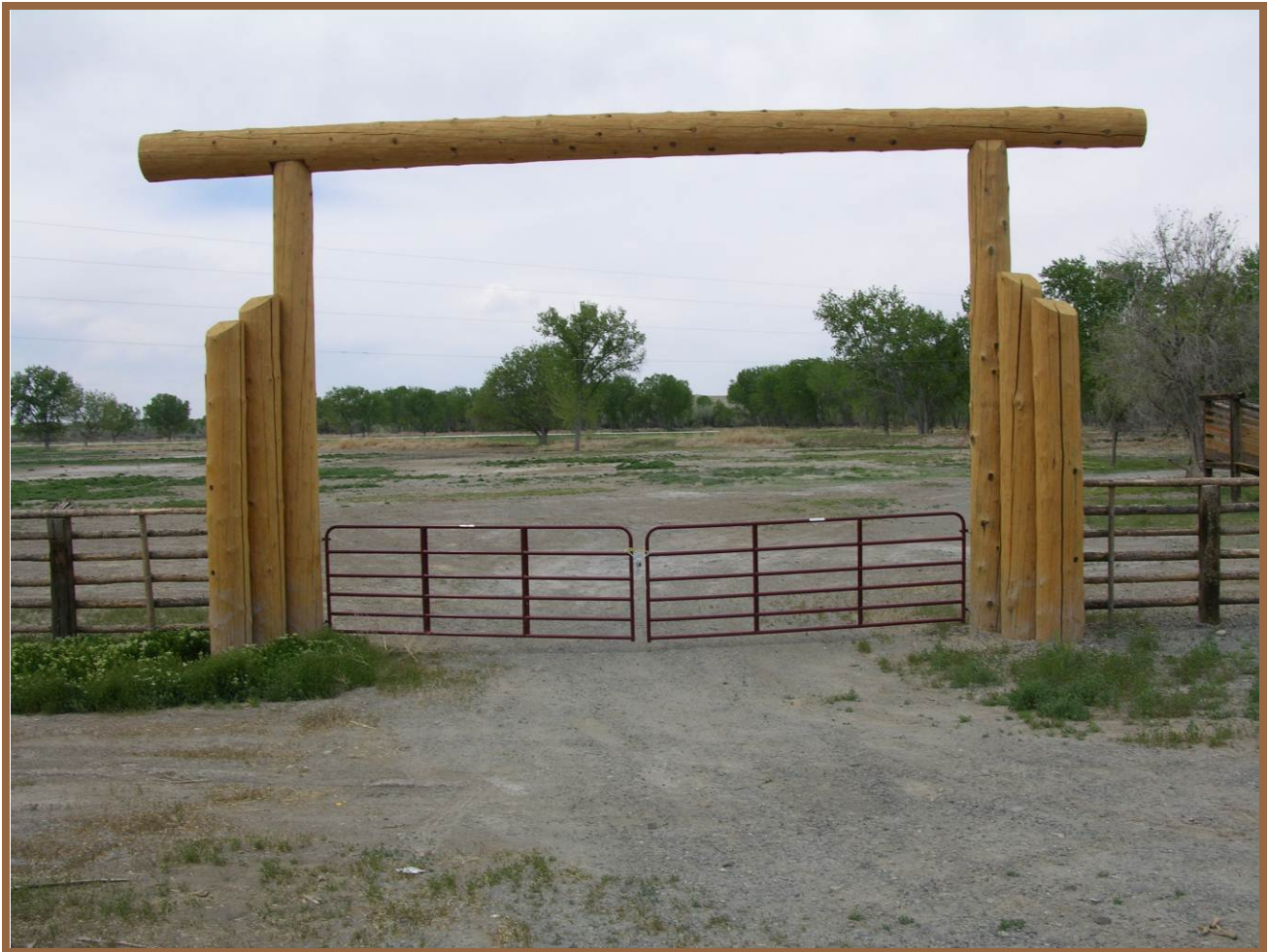
Entrance to the property lying on the west side of Highway 16.
