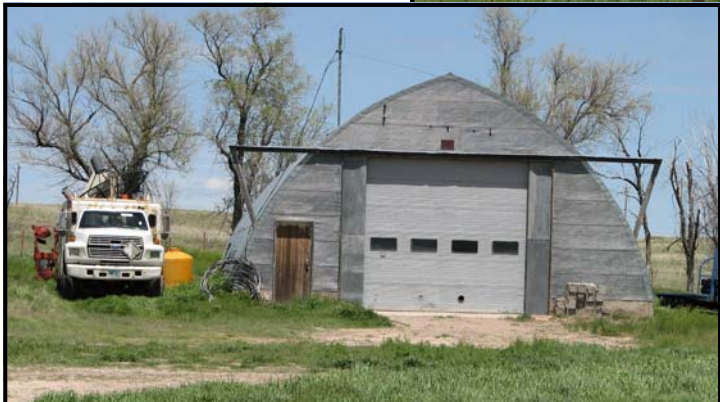
Steel Quonset with Full Cement Floor
