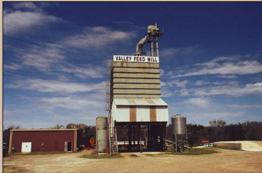
WINNSBORO FACILITY BULK LOADOUT
