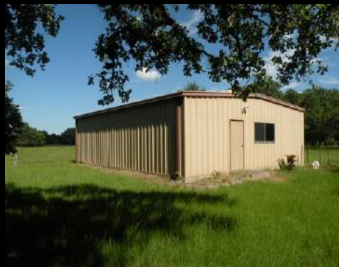
30' x 40' Insulated Barn
