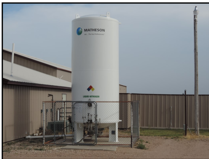
3,000 gallon liquid nitrogen tank
