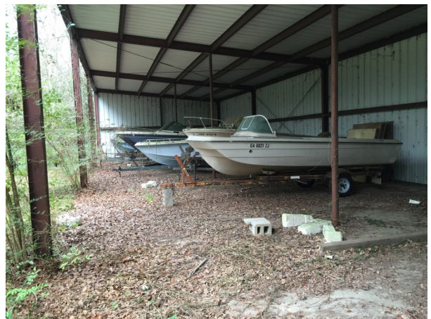
Boat Shop Shed on Concrete Pad
