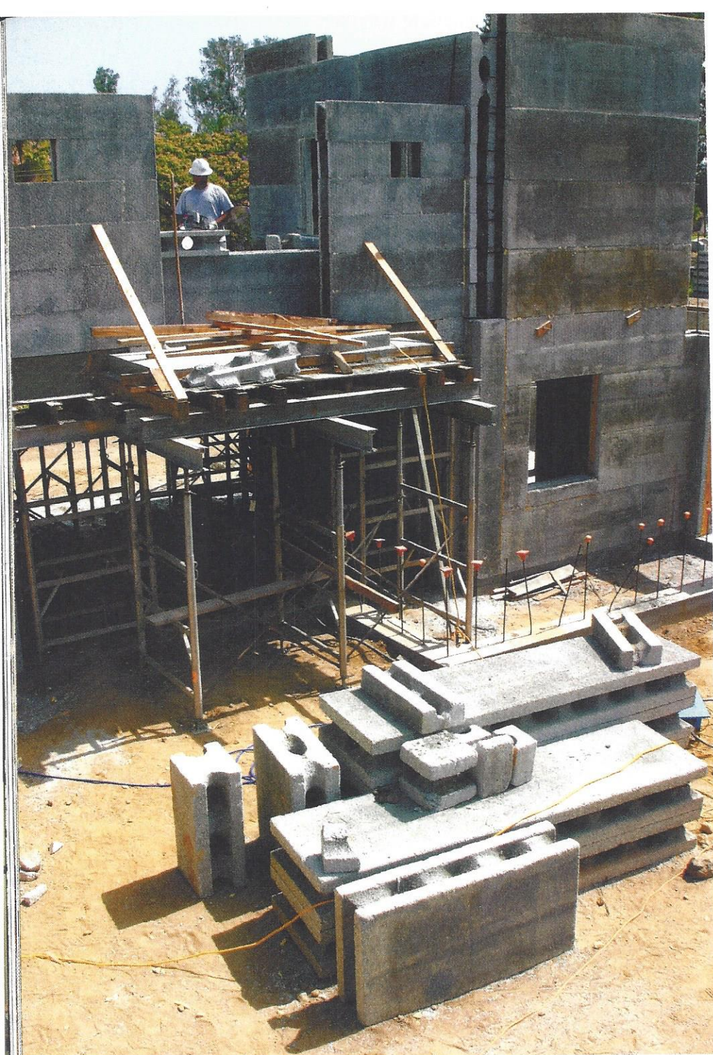
THE LARGE, LEGO-LIKE blocks are made of concrete and polystyrene, a form of Styrofoam. The building technique, popular in Arizona and New Mexico, is just gaining ground in California.
