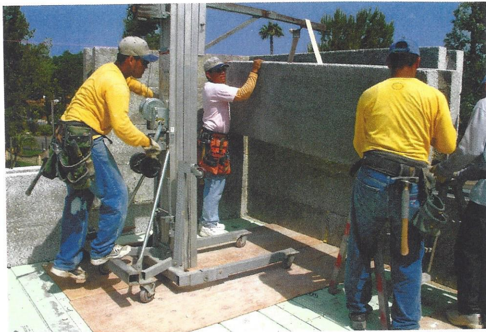
WORKERS LIFT ONE of the large sections into place on the wall. Below, they check alignment before adding mortar to solidify the sections.
