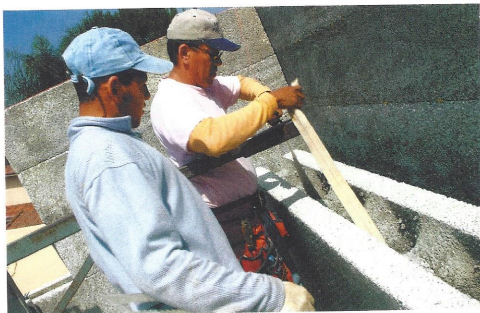
WORKERS LIFT ONE of the large sections into place on the wall. Below, they check alignment before adding mortar to solidify the sections.
