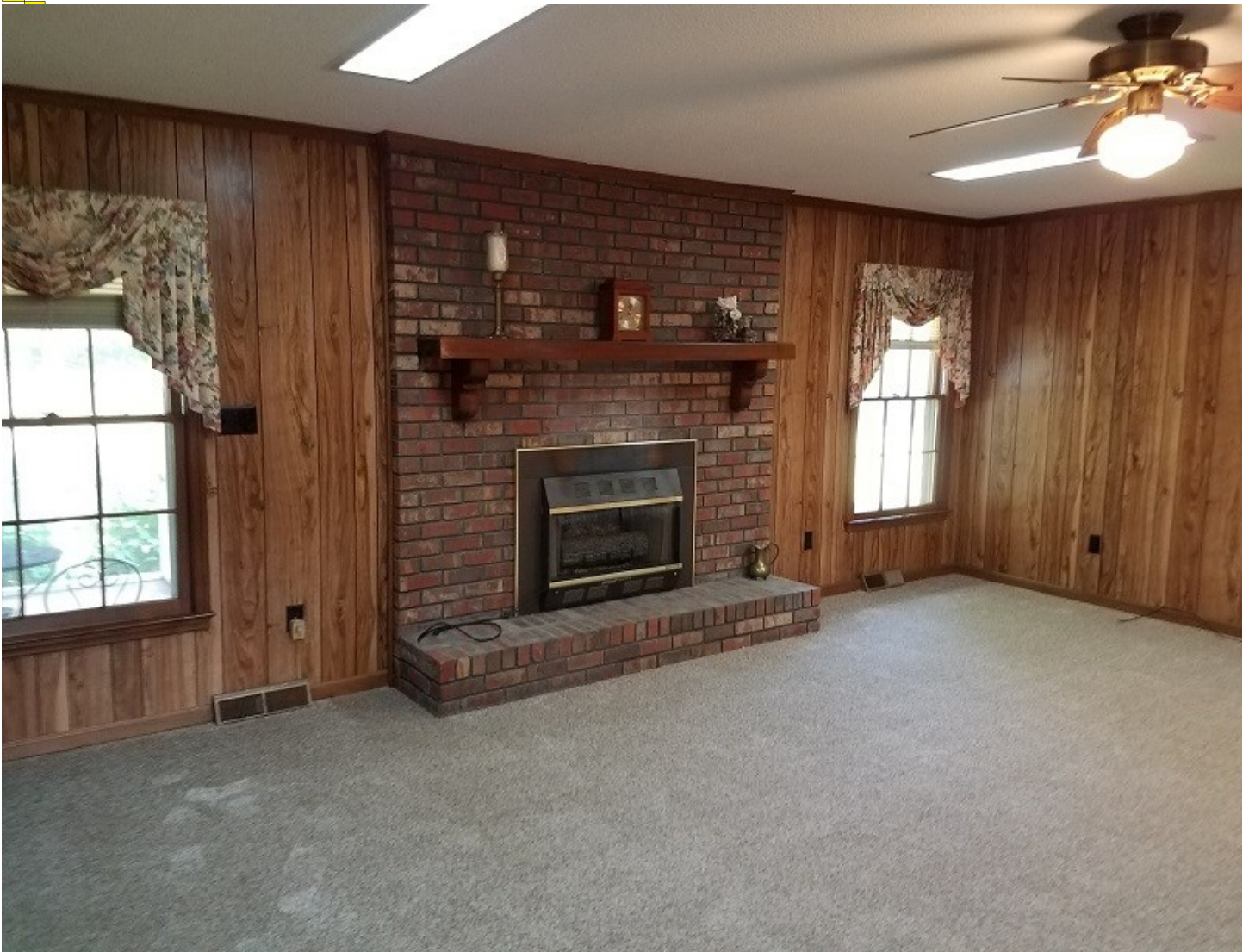
Masonry Fireplace With Insert
