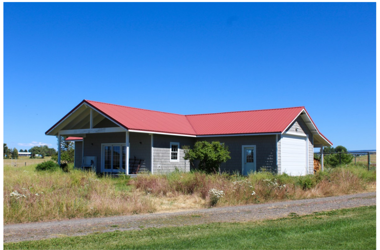
Multi-purpose building with concrete floors, a 360 sq.ft. heated shop, covered front porch, bay door and dog kennel.
