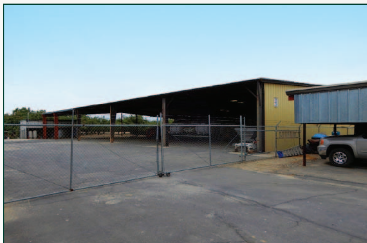
Equipment storage building
