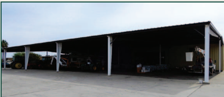
Equipment storage building
