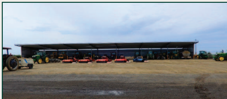
Equipment storage building
