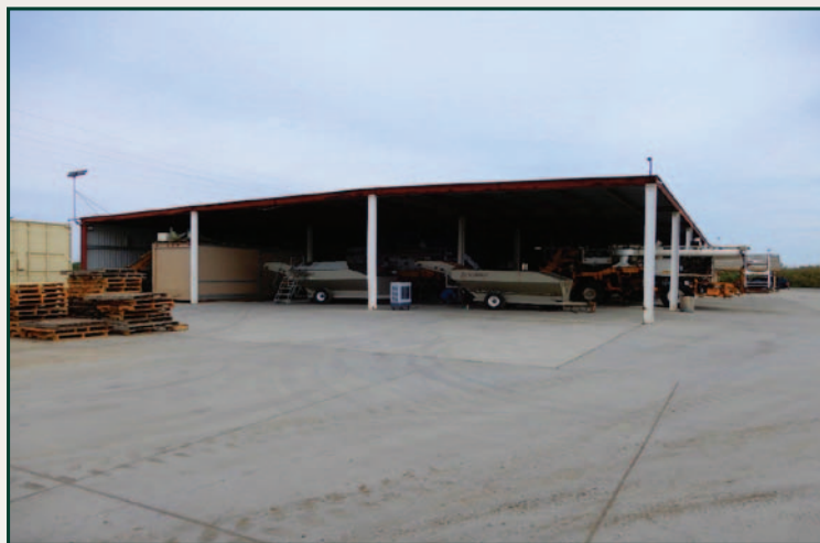
Equipment storage building
