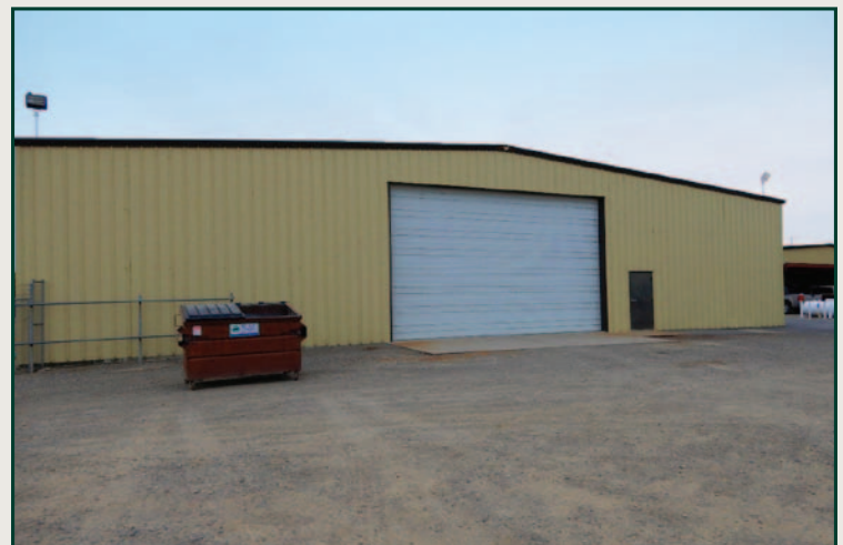
Equipment storage building
