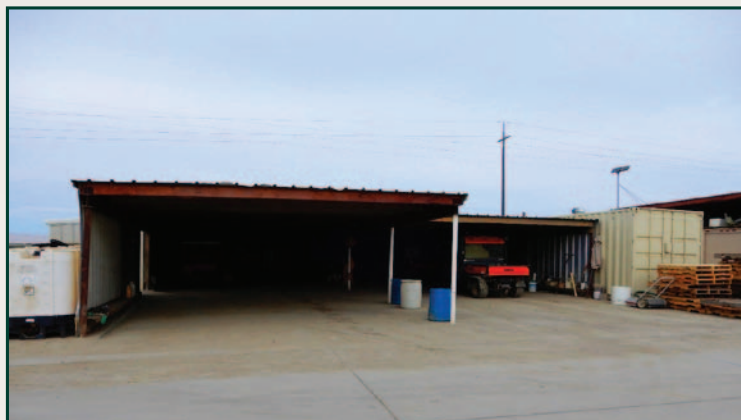
Equipment storage building
