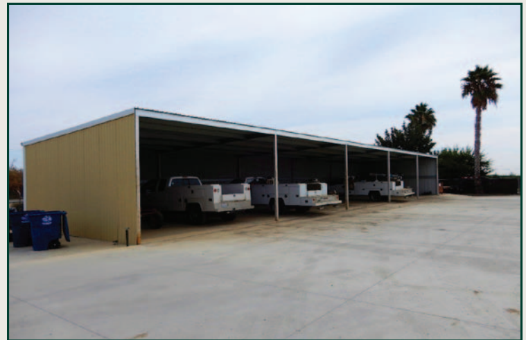
Equipment storage building
