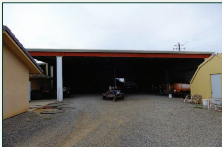
Equipment storage building
