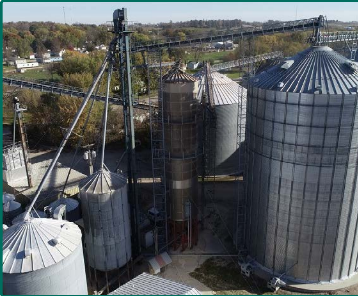
Grain Dryer & Bins
