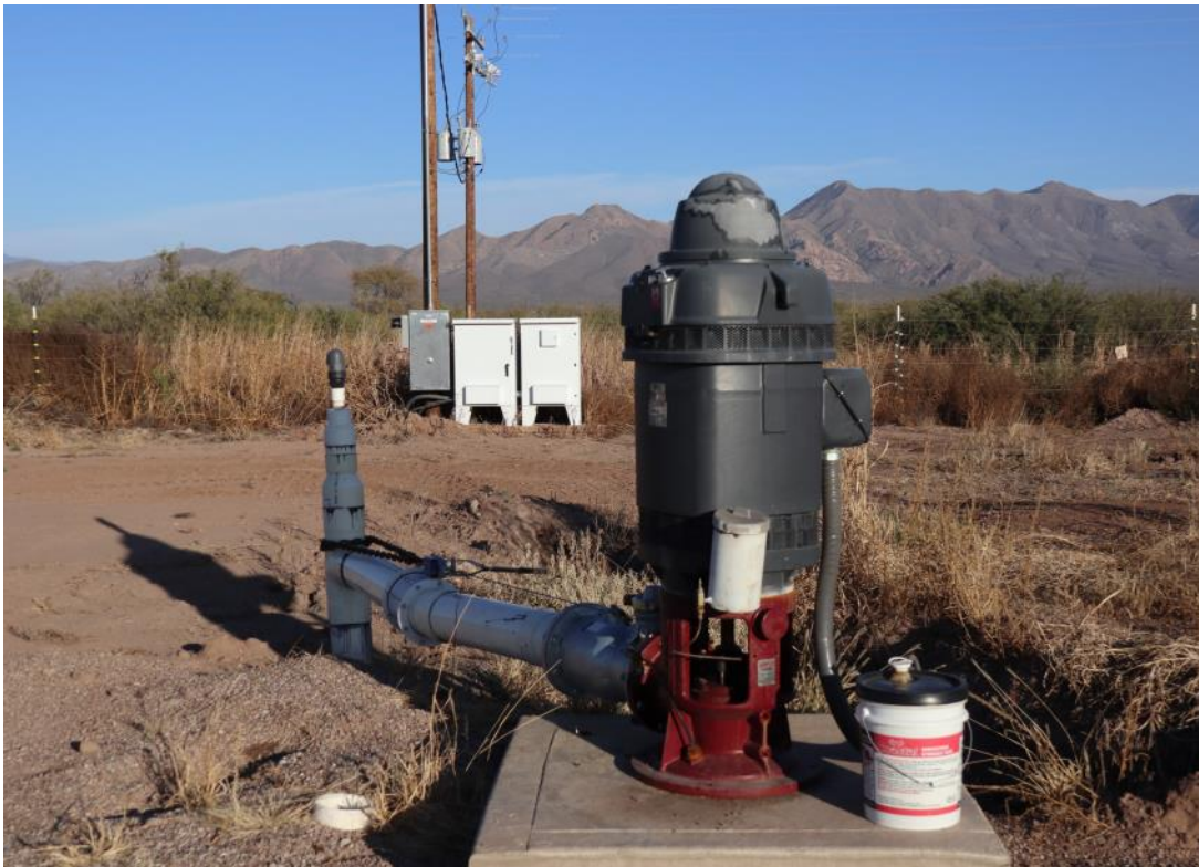
Well 1,005' deep, 12 3/4" casing, 150 hp, 600 –650 gpm
