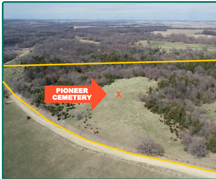
South Looking North
