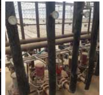
Main hot water pumps for radiant heat
