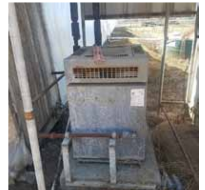
Heat exchanger from steam to hot water.
