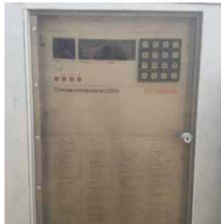
Computer control system, for heat, humidity, irrigation, and greenhouse ventilation
