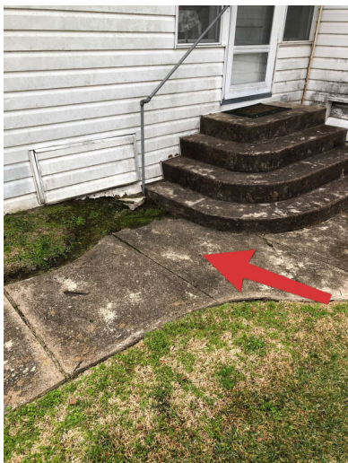
Slope towards crawlspace
