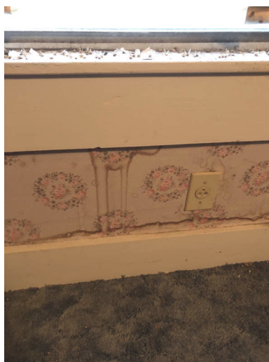
2nd Floor Bedroom: no elevated moisture content at time of inspection
