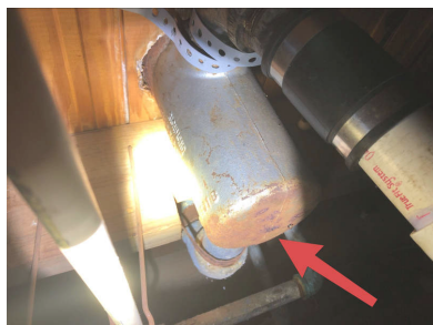
2nd Floor Bathroom: cannister trap
