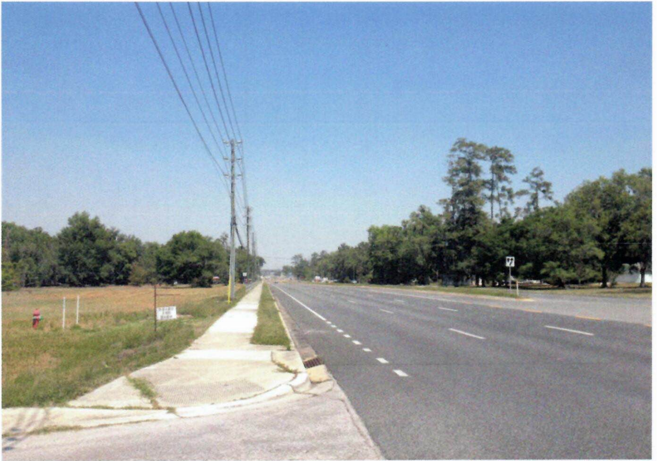
Facing South along US 41
