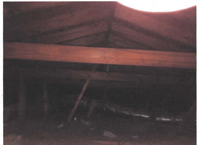
Site Built Roof Framing
