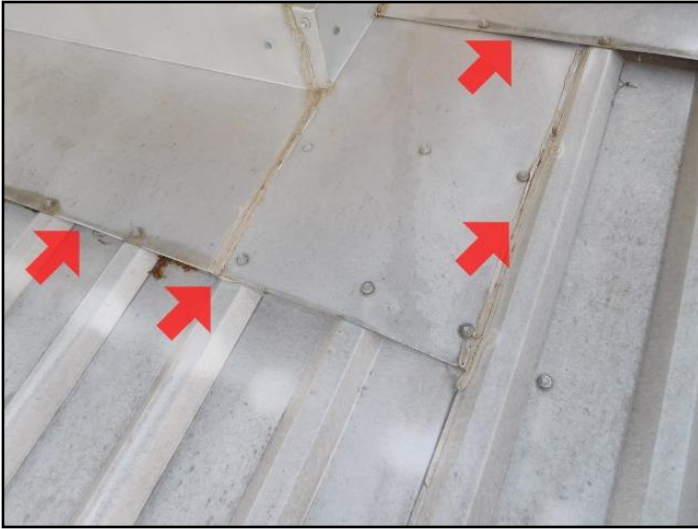
40. deteriorated caulking around flashing
