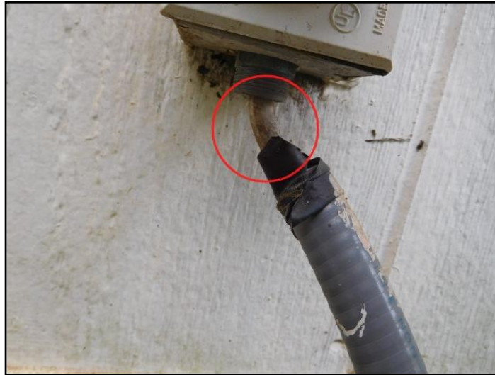
17. Wires not well secured to outlet box
