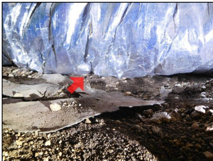
21. ductwork laying on the ground
