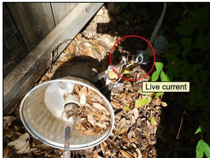
16. Wires not well secured to walls
