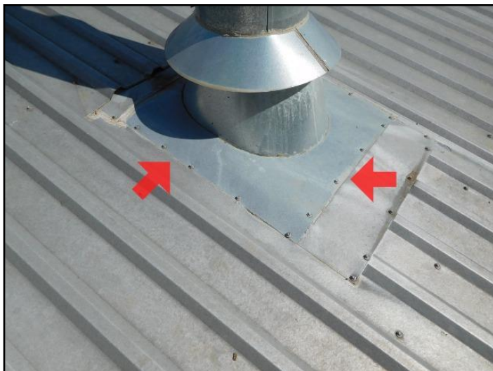
38. deteriorated caulking around flashing
