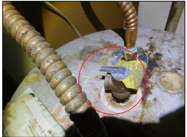
29. Discharge tube missing
