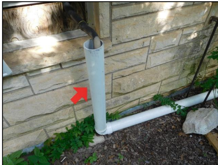
83. Washing machine waste pipe
