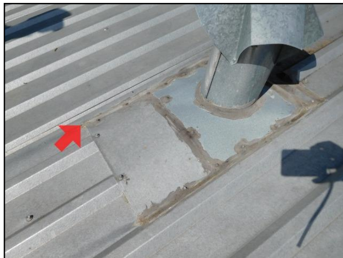
39. deteriorated caulking around flashing
