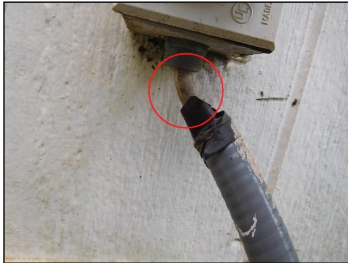
62. Wires not well secured to outlet box
