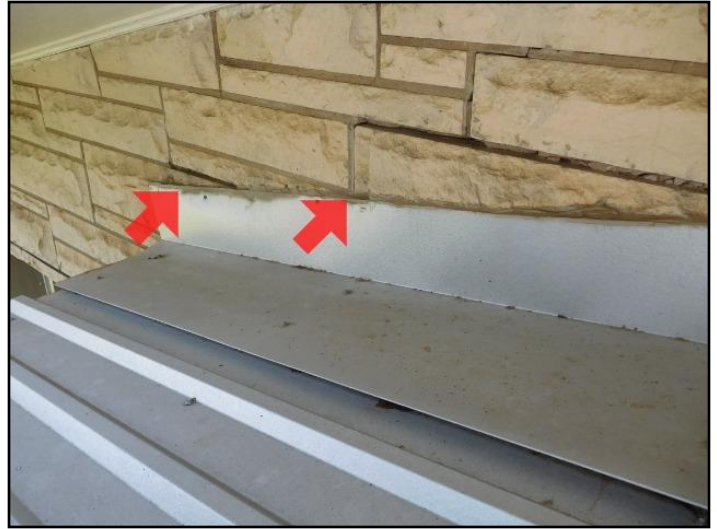
41. deteriorated caulking around flashing
