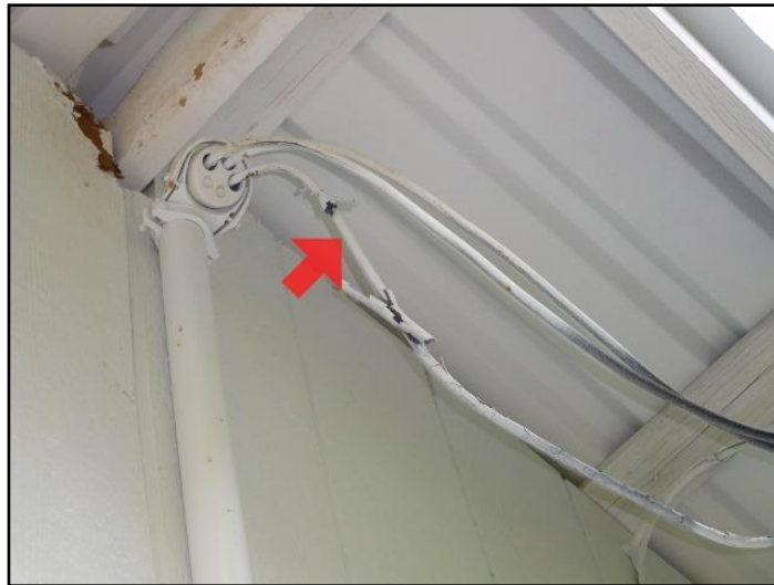
5. Insulation missing or damaged
