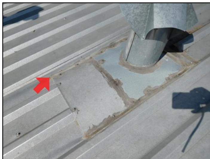
2. deteriorated caulking around flashing
