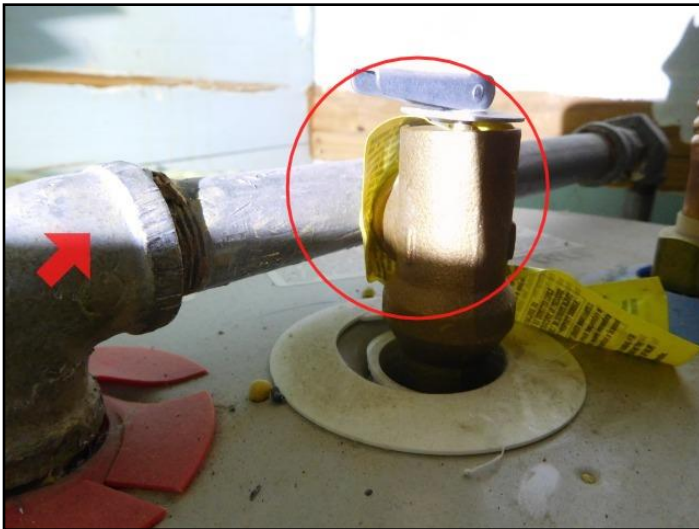
28. Discharge tube missing
