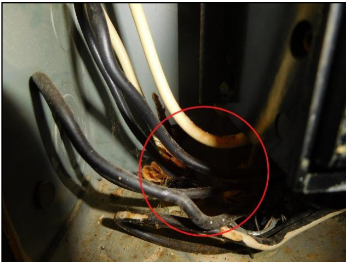
54. Ungrounded wiring - cloth
