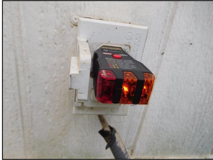
60. No GFCI/GFI (Ground Fault Circuit...
