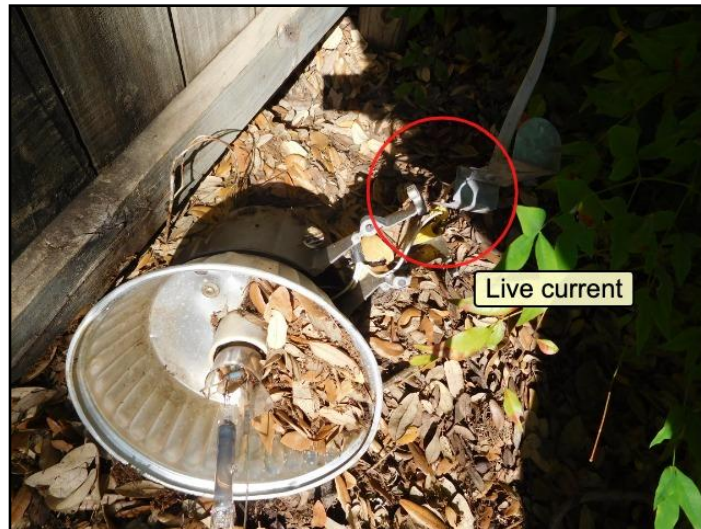
59. Wires not well secured to walls
