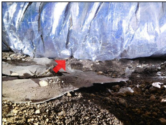
68. ductwork laying on the ground
