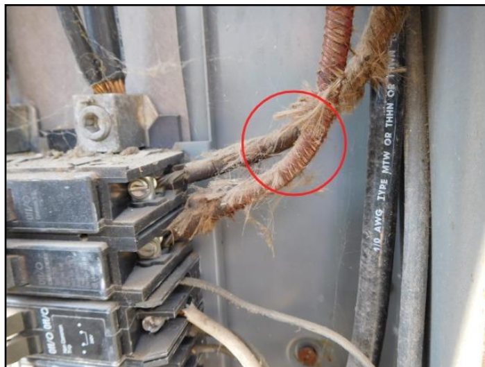
9. cloth aluminum wiring
