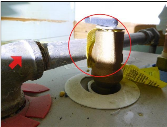
80. Discharge tube missing
