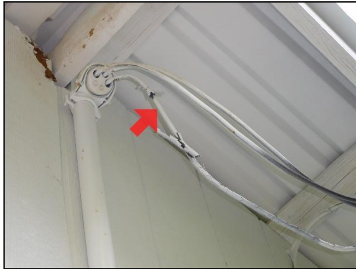
48. Insulation missing or damaged
