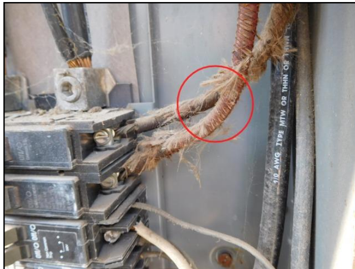
51. cloth aluminum wiring
