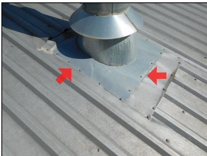
1. deteriorated caulking around flashing
