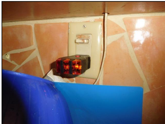
61. No GFCI/GFI (Ground Fault Circuit...
