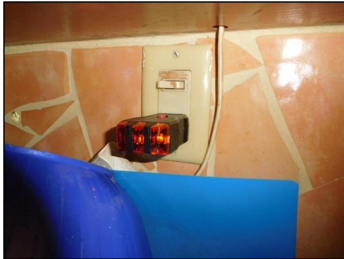
19. No GFCI/GFI (Ground Fault Circuit...
