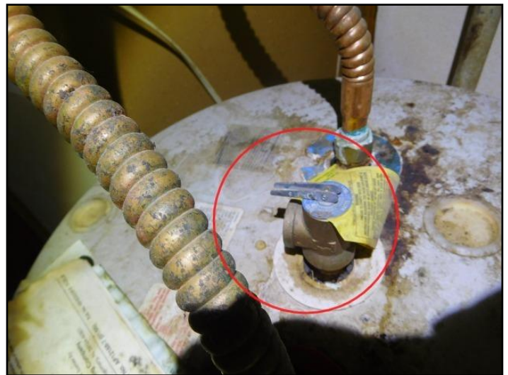
81. Discharge tube missing
