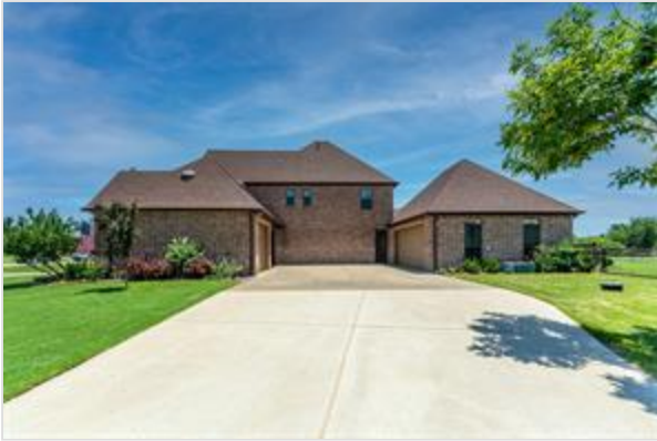
SIDE OF HOME...View Of Concrete Drive, 2 Car Garage And Single Car Garage
