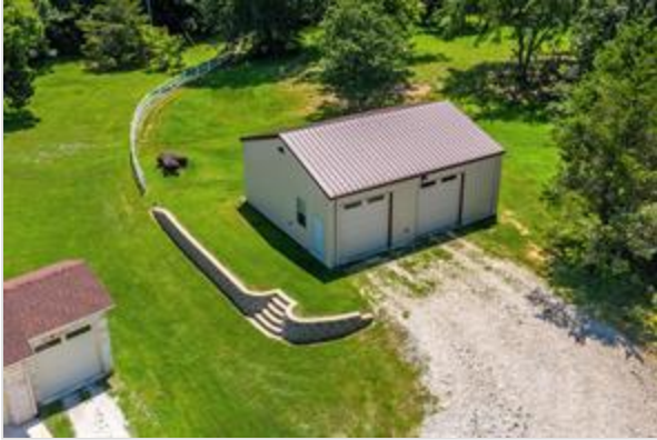
WORKSHOP...Approx 30x36, Foam Insulated, Concrete Slab, 2-10x10 Auto Overhead Doors And 1 Walk-Thru Door
