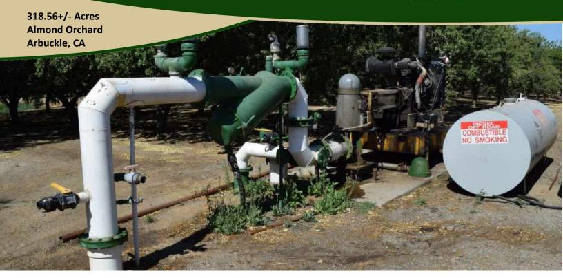
2nd well is diesel with a spin-clean filter
