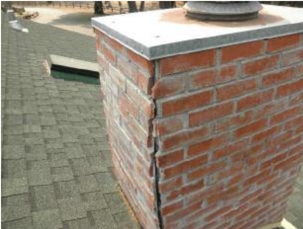
The faux brick veneers around both of the chimney enclosures are loose/separated.
