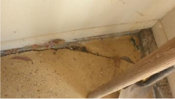
Settlement crack at the SW corner of the garage.
