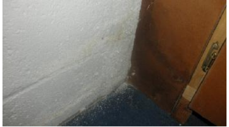
Evidence of water intrusion at the CMU block wall/cabinets in the basement
