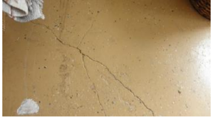
Settlement crack at the SW corner of the garage.
