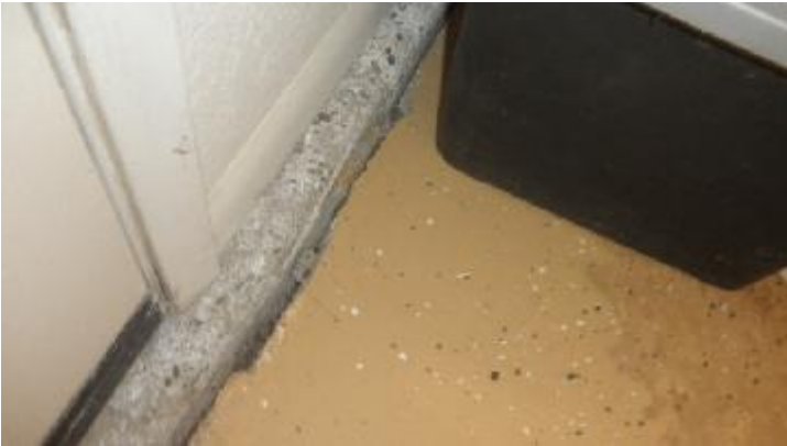
Slab pulled away from the stem wall at the west side of the garage.
