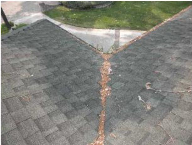
Clean the debris off the roof.
