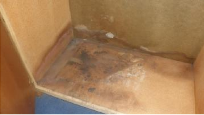
Evidence of water intrusion at the CMU block wall/cabinets in the basement
