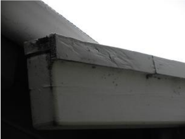
Moisture damage at the wood siding and trim at the half bathroom.
