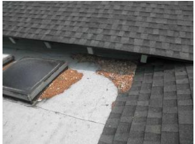
Clean the debris off the roof.
