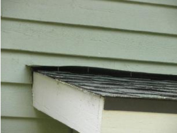
The roof-to-wall flashing above the master bedroom is uplifted.
