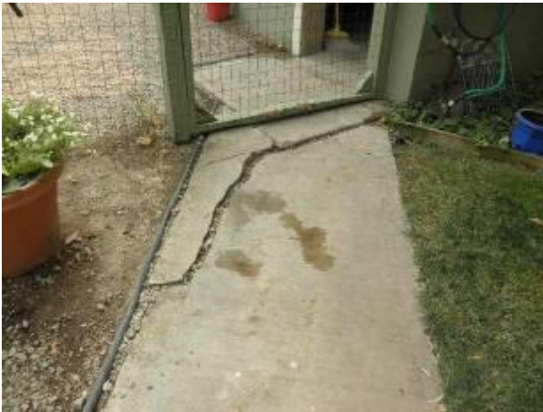
Large crack in the concrete walkway.
