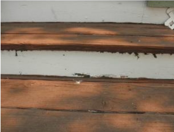
Moisture damage to parts of the exterior landing.
