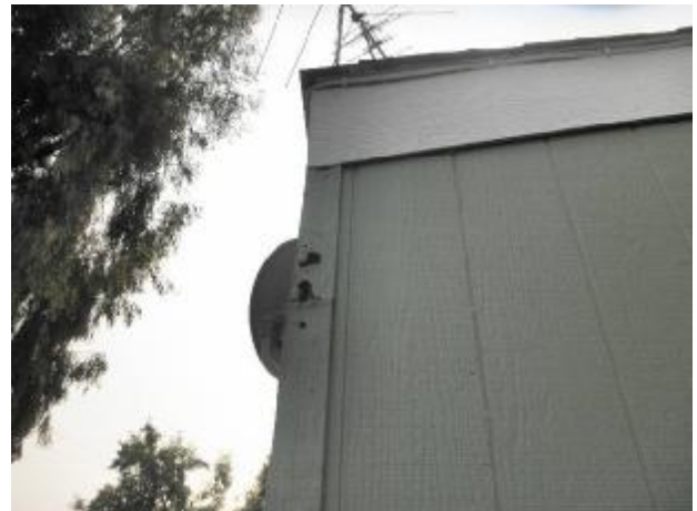
Moisture damage at the corner wall trim.
