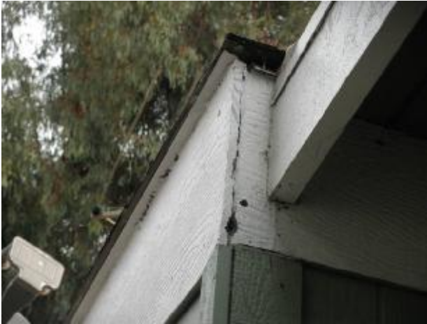
Moisture damage at the fascia board.
