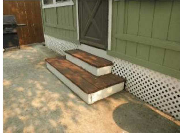
Bottom step riser exceeds the max allowable height of 7 3/4"
