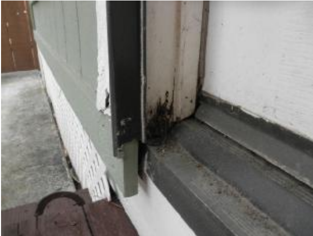
Moisture damage to the base of the jamb at the exterior door on the west wall of the family room.
