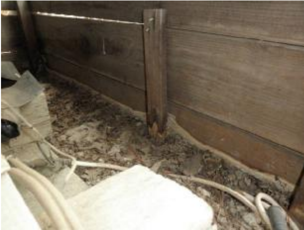
Fungus damage to parts of the perimeter skirting.
