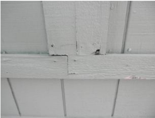
Moisture damage at the wall trim.
