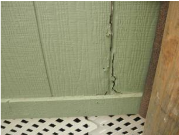
Moisture damage at the wood siding.
