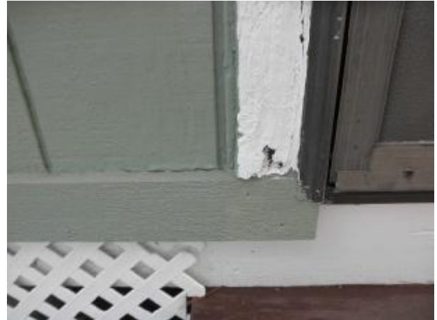
Moisture damage to the door trim.
