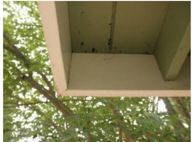
Moisture damage at the eave.
