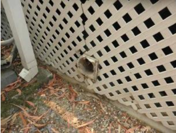
The dryer lint exhaust vent hood is damaged.
