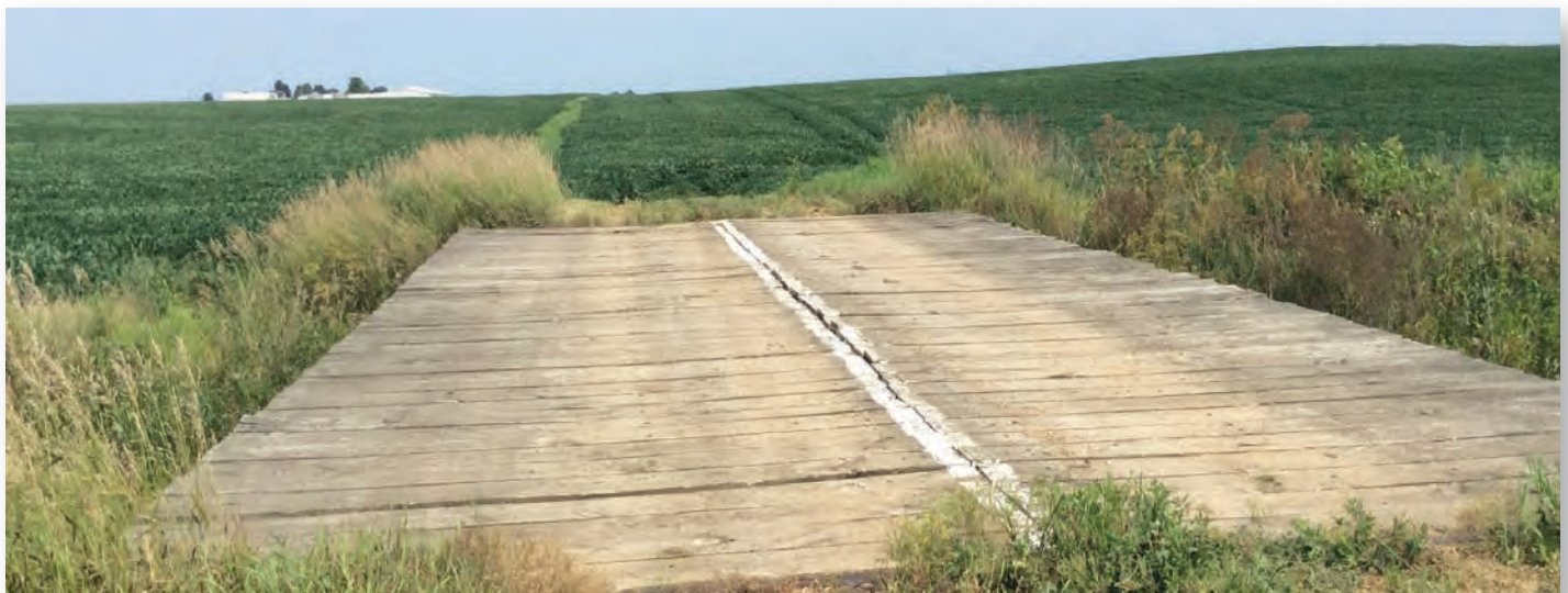
looking east from bridge, 7.27.21
