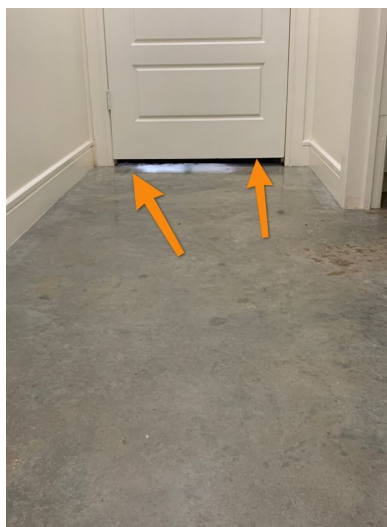
Missing threshold to seal garage to living area
