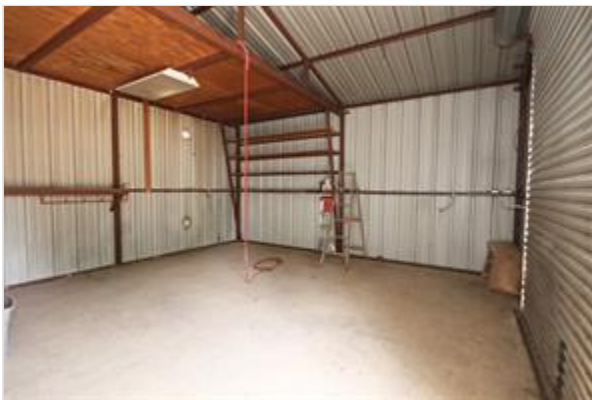
WORKSHOP/STORAGE BLDG INTERIOR
