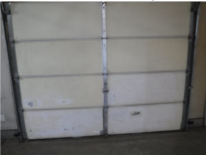
Minor damage noted on the insulation panels and the exterior panels
