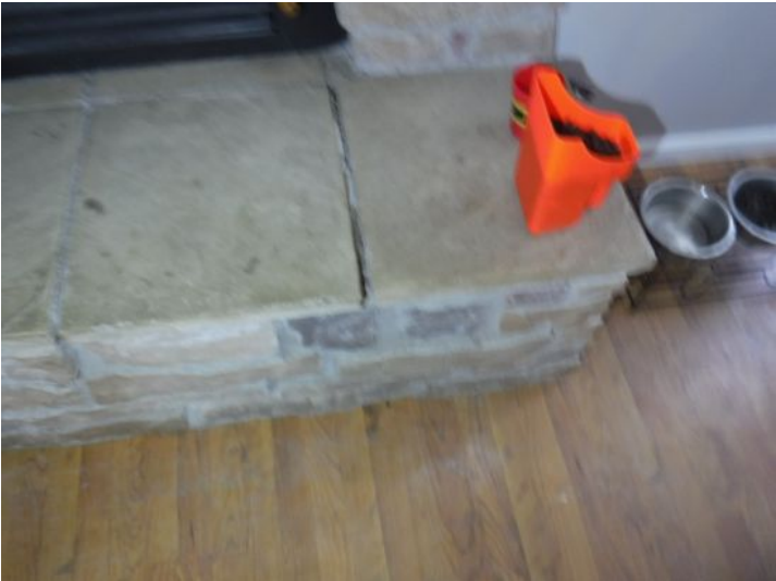
The mortar needs to be repaired on the stone hearth
