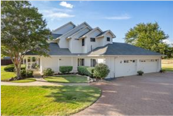
Three car garage and a stamped concrete driveway.
