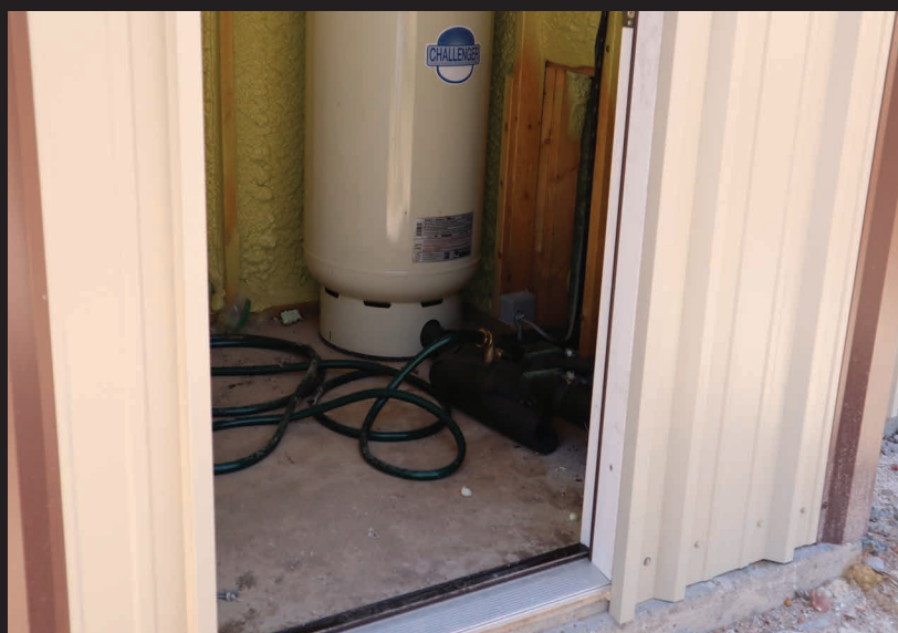
Tract 1: 2021 Drilled Well. 340ft Depth. Yield is 15gpm
