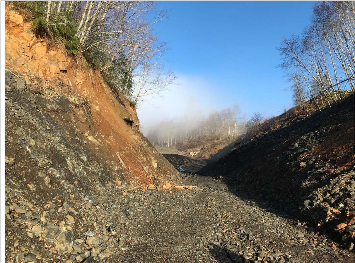
Photogrpah 2: The water impoundment overflow outlet is to an area of blast rock for groundwater infiltration.
