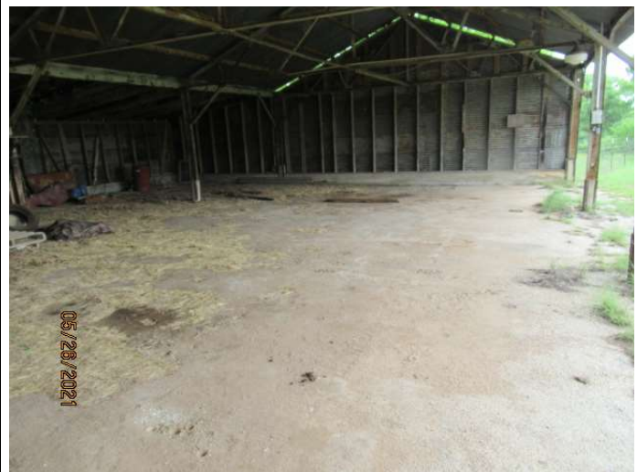
View beneath overhead shed located west of home.
