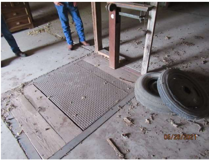
Scale observed inside the warehouse.
