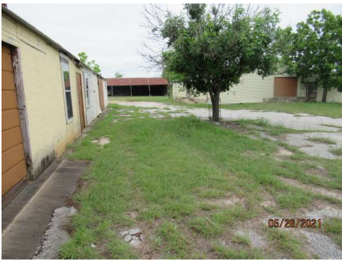
Former sprayer shop located west of home.
