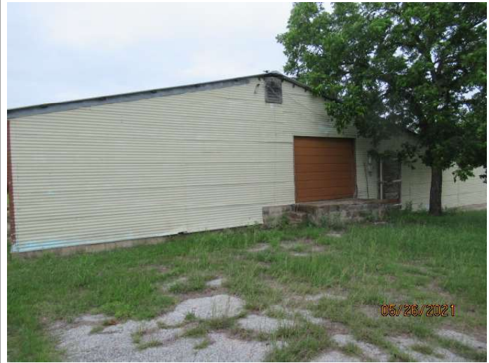
View of east side of chemical warehouse.
