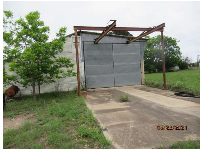
View of west side of vacant shop.
