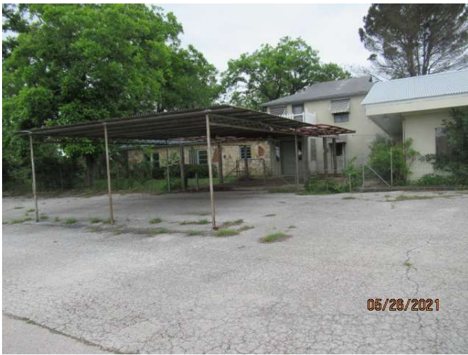
Front entrance into home under the metal canopy.
