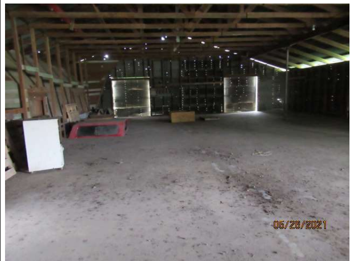
Interior view former chemical storage warehouse.
