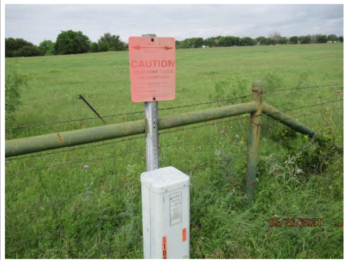
Telephone cable warning post located on north side.
