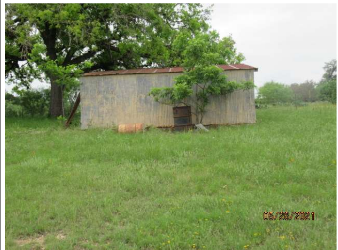
Storage shed located south of sprayer shop.
