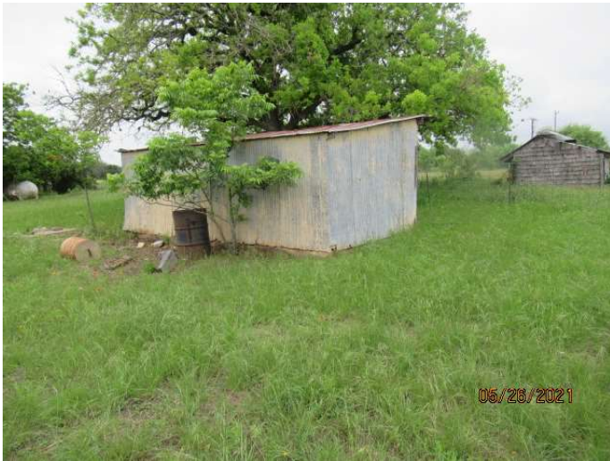
Storage shed observed on west side of property.
