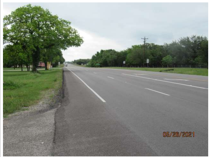
Viewing east along US Highway 290.
