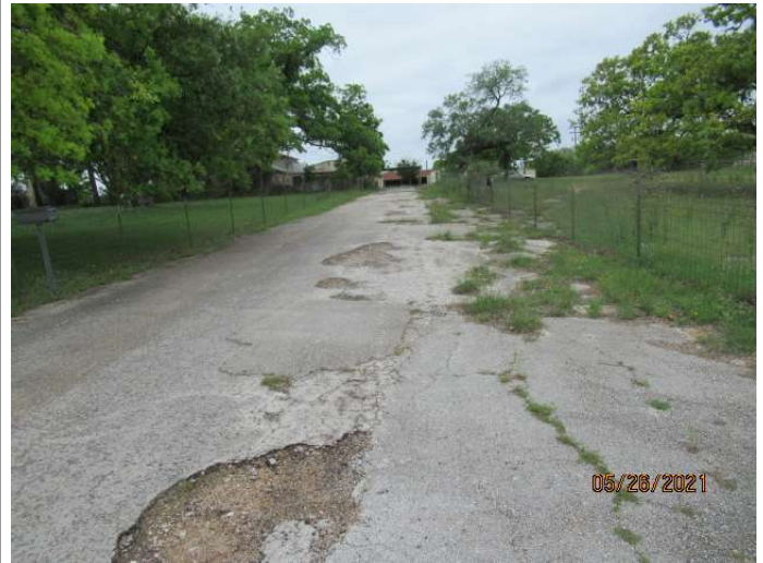
Driveway to home and buildings via Elberta Street.
