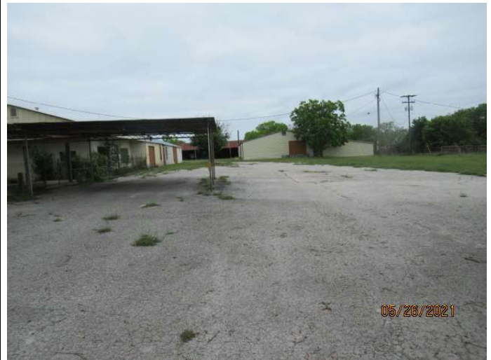
Parking area and canopy observed on the property.
