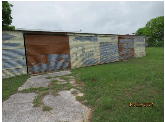
View of north side of the warehouse.
