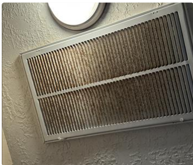
Air return vent first floor, visual microbial growth
