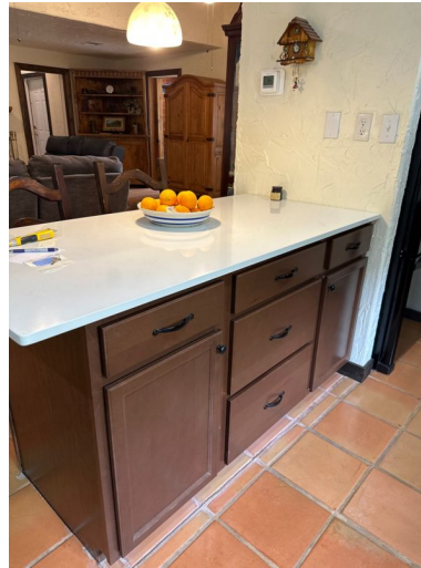
No GFCI protection found on the kitchen island
