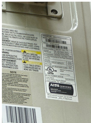
Cooling Condenser Unit #2: Electric Condensing Unit, Heat Pump, Mini split
