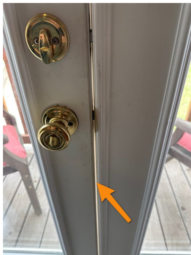
Daylight between the French doors right front second level bedroom
