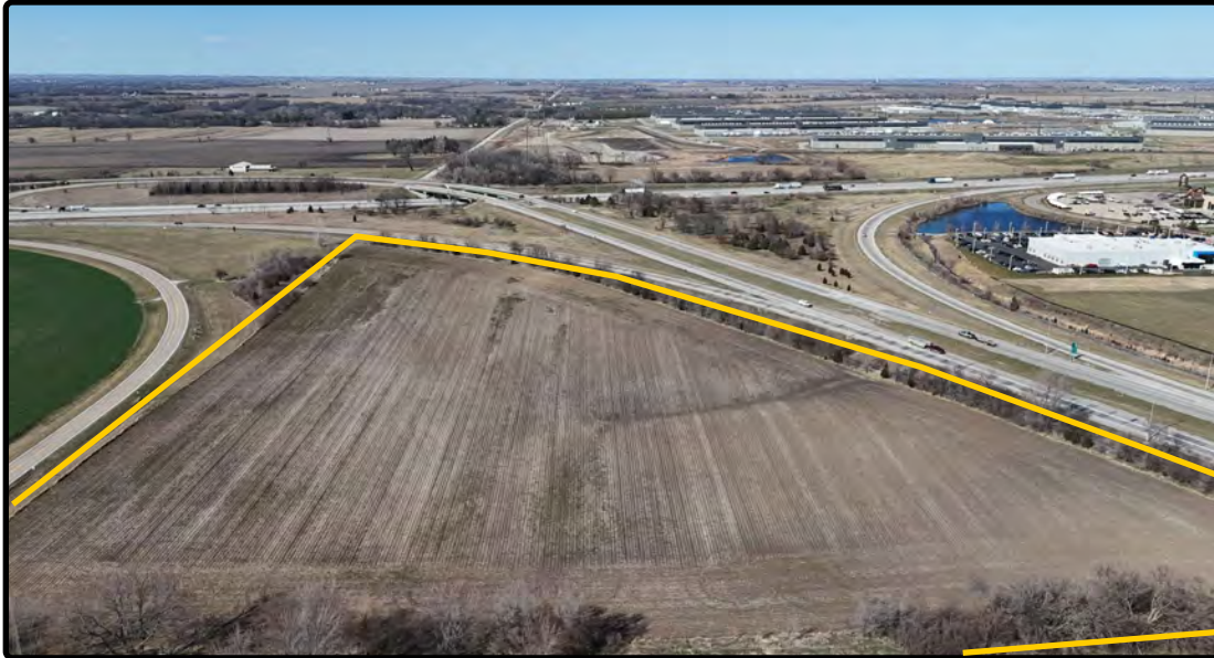
South Looking North
