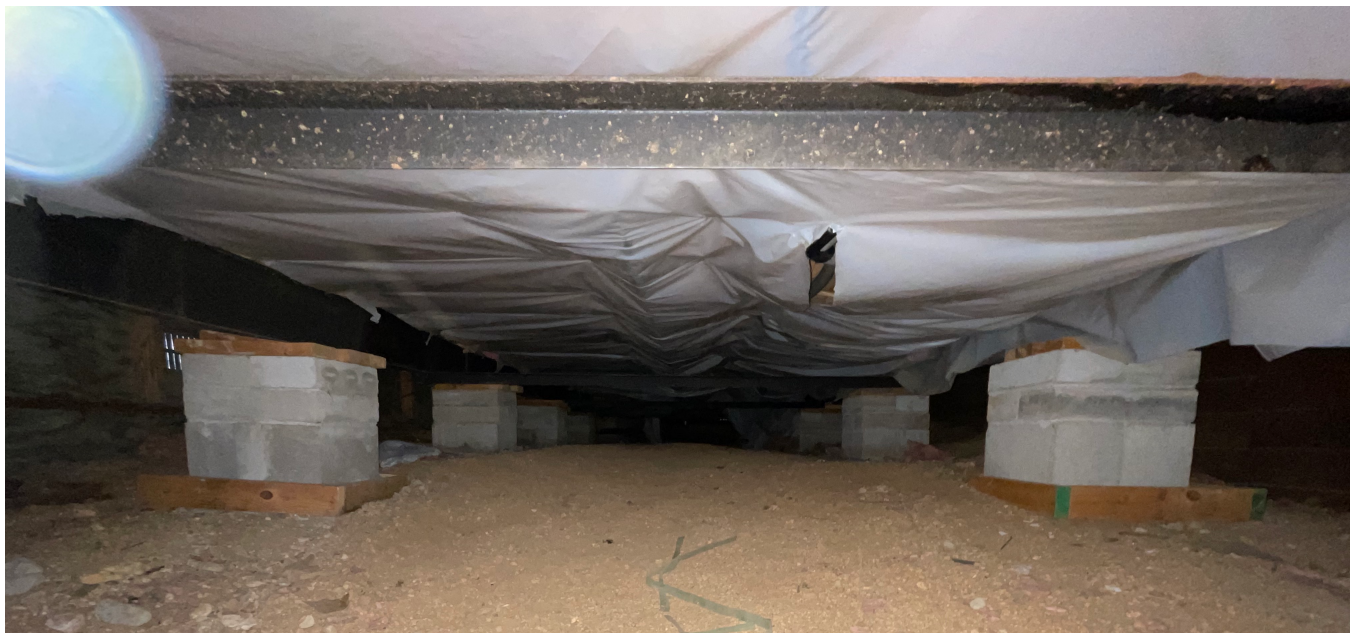
Figure 1, CMU Pier Support Foundation
