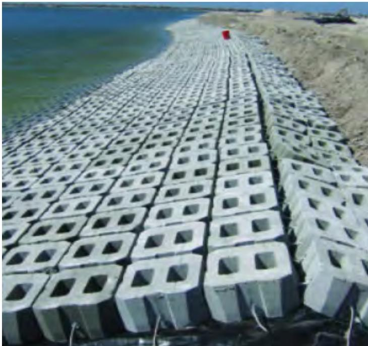
**Figure 5. Articulated Concrete Blocks Example (Acfenvironmental.com)**
