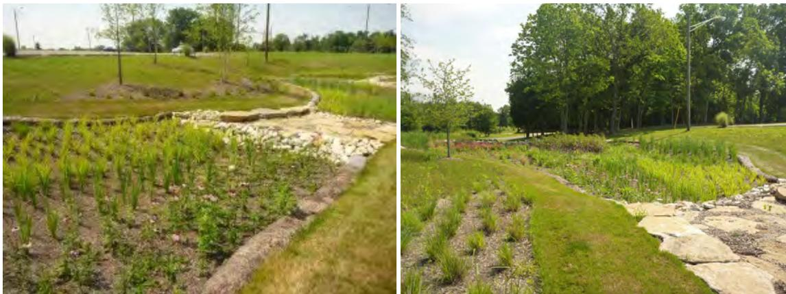
**Figure 124. Bioretention Basins (stormwater.wef.org)**
