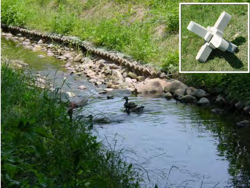
**Figure 7. Example of A-Jack Revetment (conteches.com)**
