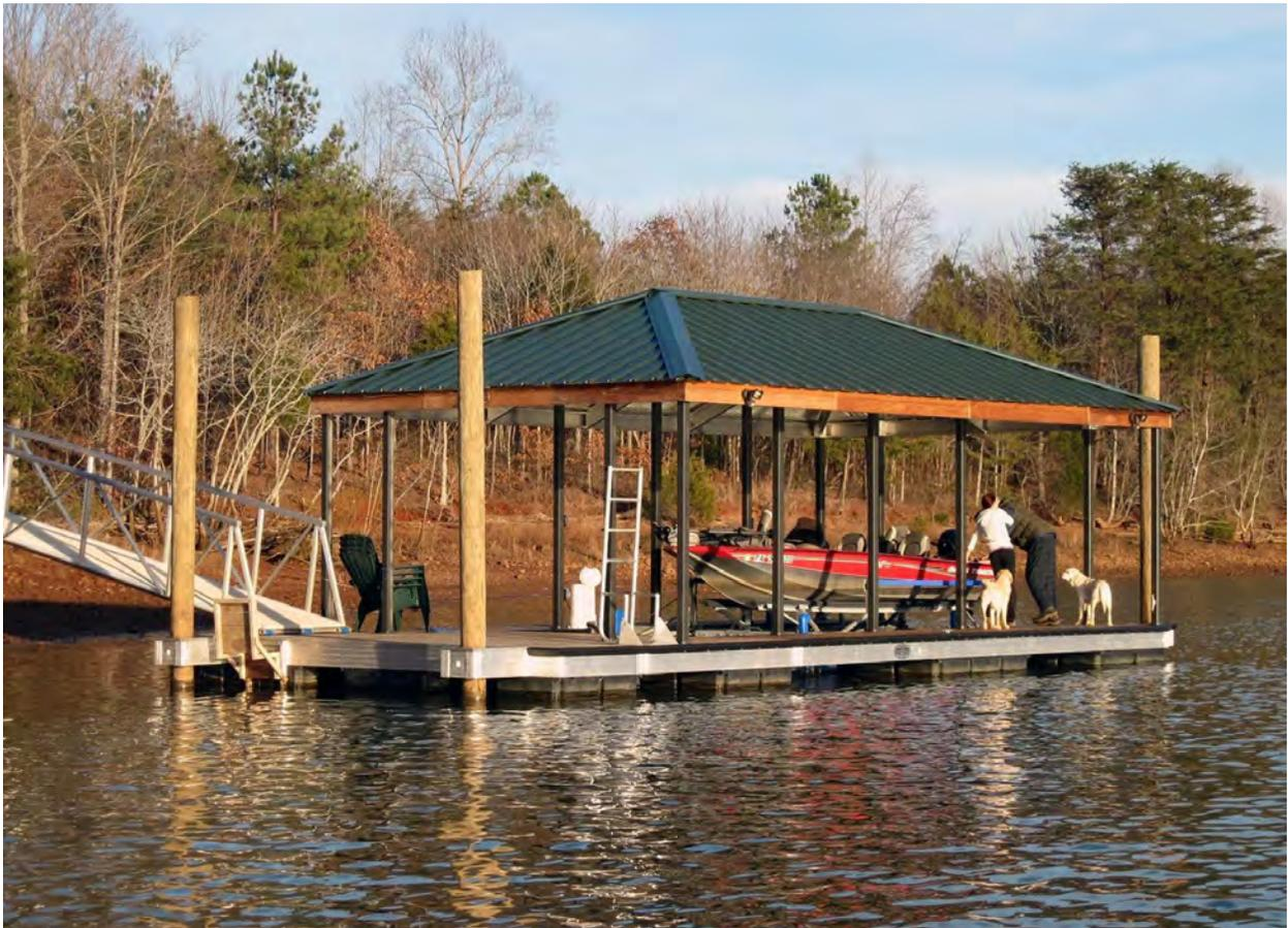
**Figure 2. Example of Floating Pole Dock**
