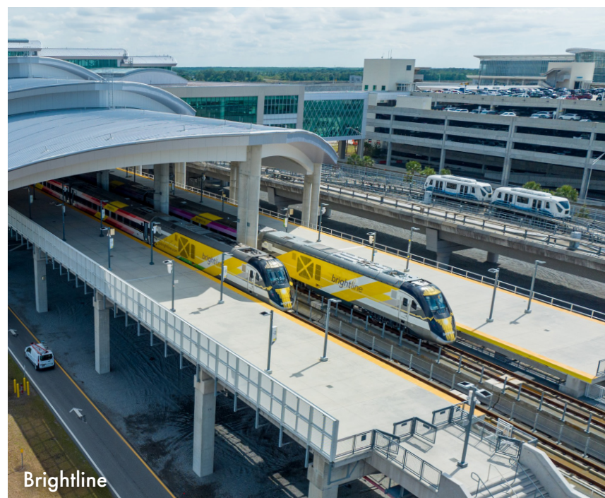
Orlando International Airport
