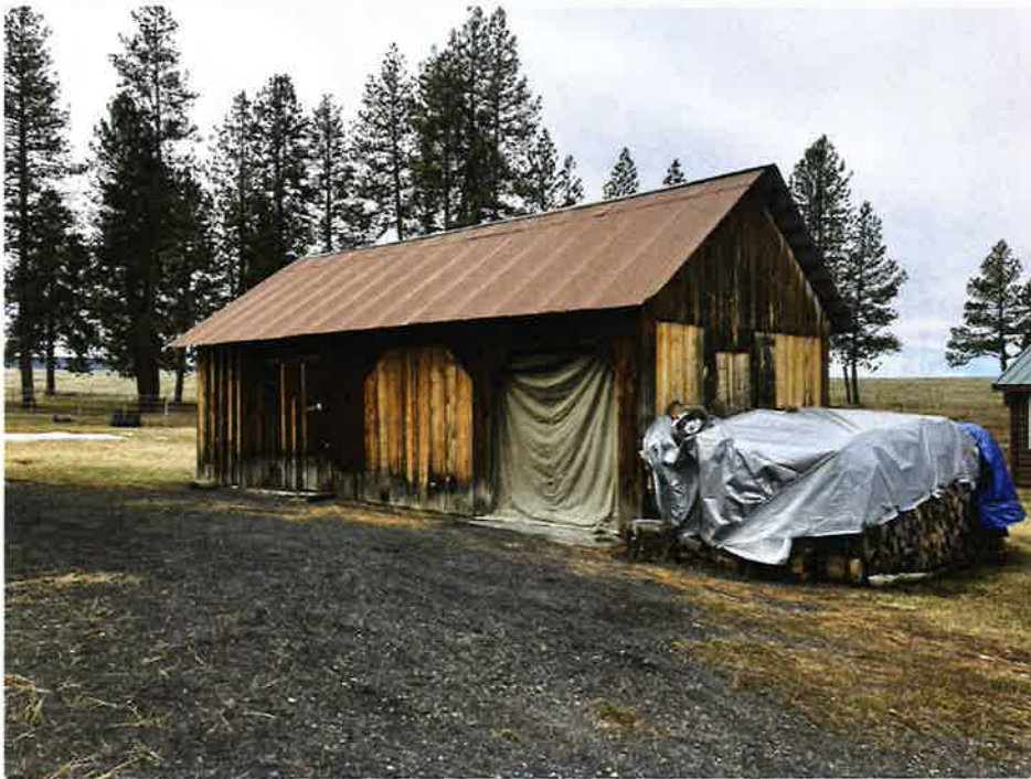
Machine and tool shed with pine siding
