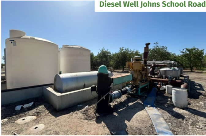
Diesel Well Johns School Road
