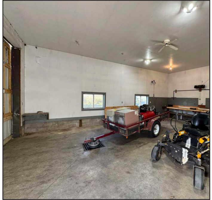
Interior of Utility Building
