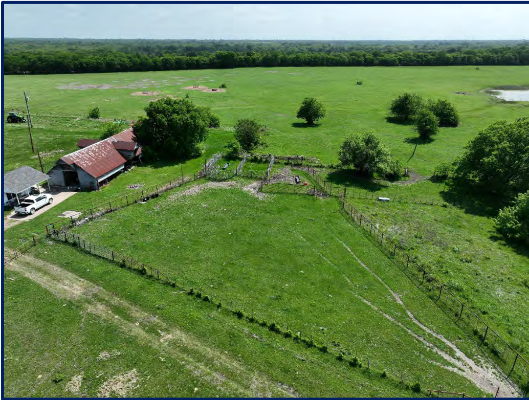
View of the steel pipe cattle pens and old 2,400 square foot wood frame barn.
