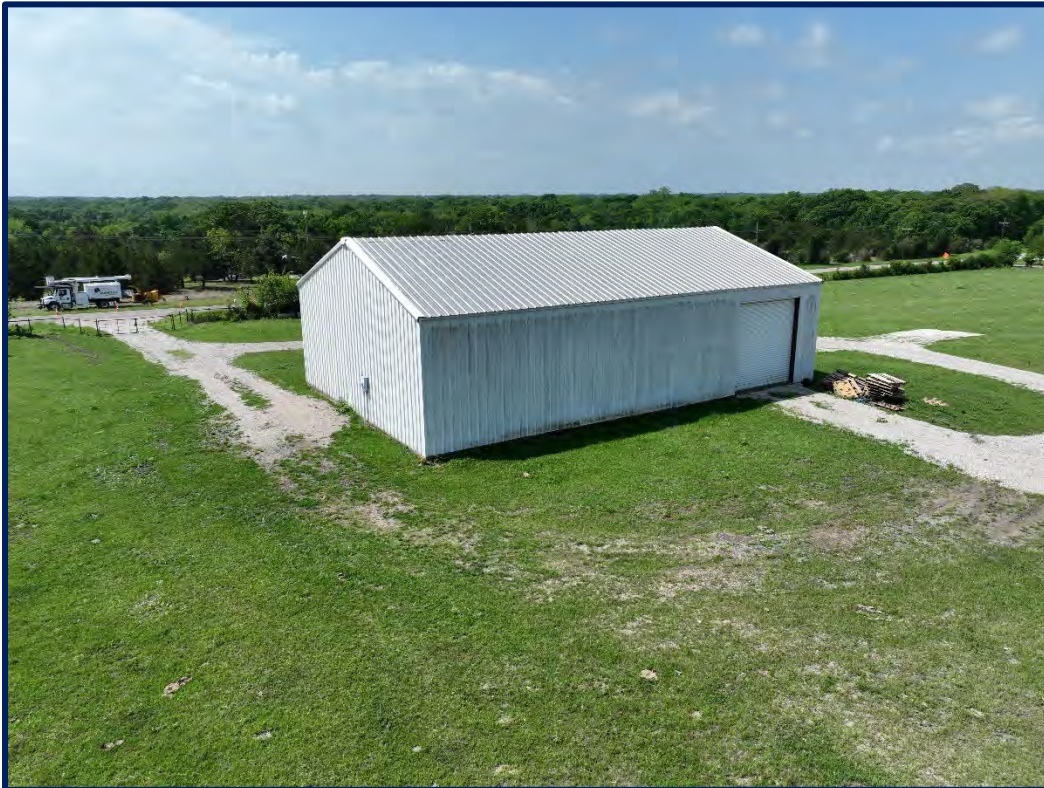
2,400 square foot shop located in the southwest part of the east tract.
