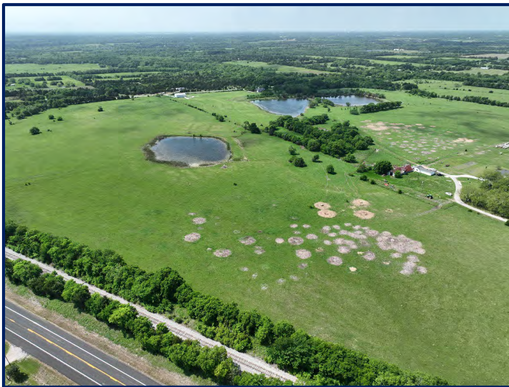
Southwesterly view from above US 69 and the Dallas Garland & Northeastern Railroad.
